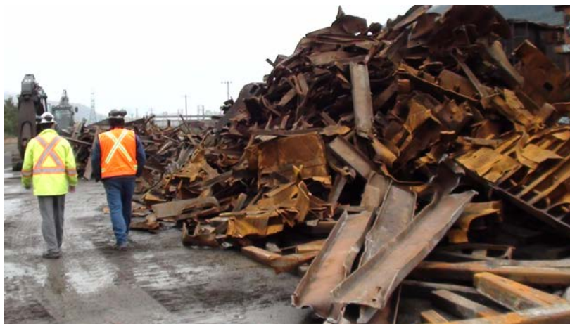
Viewing of the metal salvage and sizing facility
