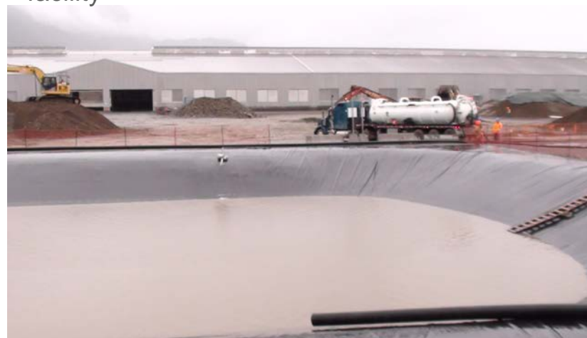
Viewing of one of 5 construction water ponds
