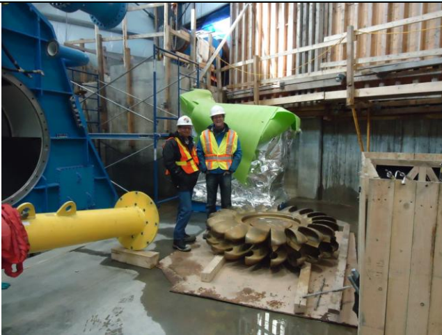
The Powerhouse: 1 of 4 turbine runners installed
