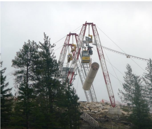
Cable Crane: bringing construction materials and personnel over the Fraser River - one piece at a time.
