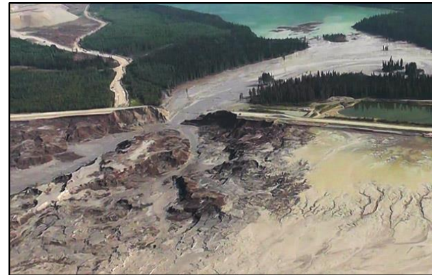
Mt Polley tailings pond breach
