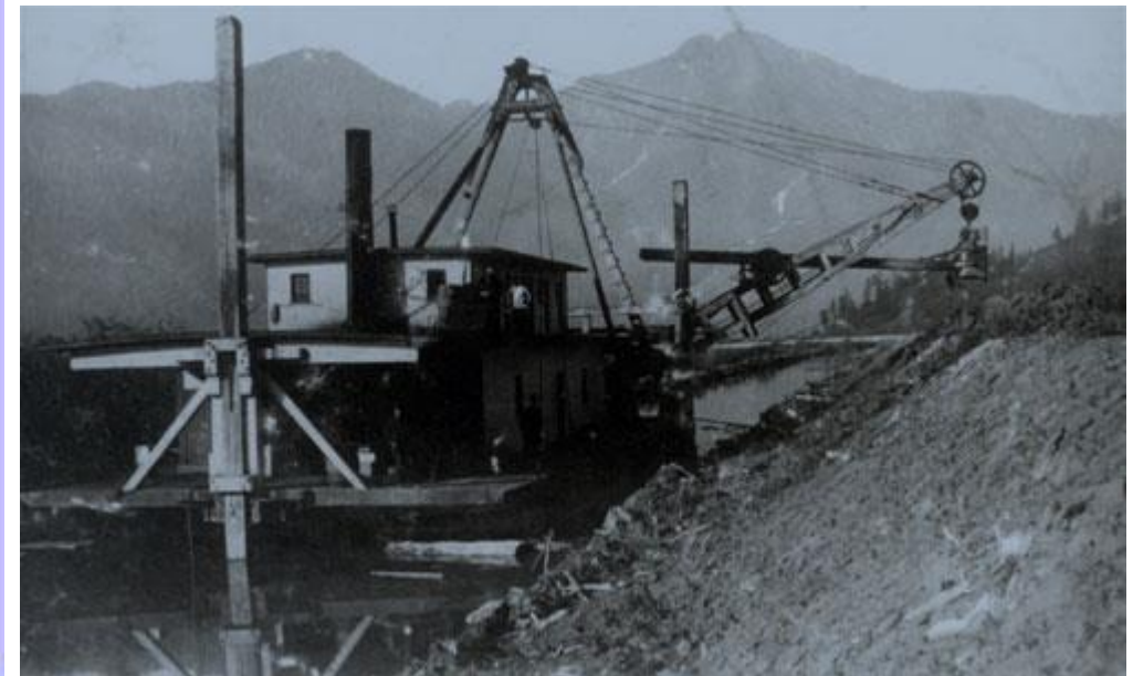
Electric dragline building up the dyke on the Vedder Canal.
